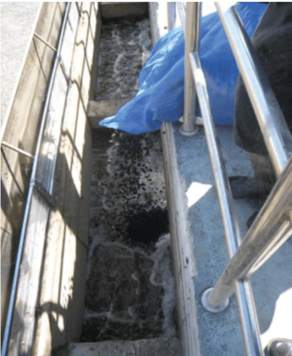
**Fig 2: Filling of Levapor MBBR IFAS media in the Aeration Tanks**
